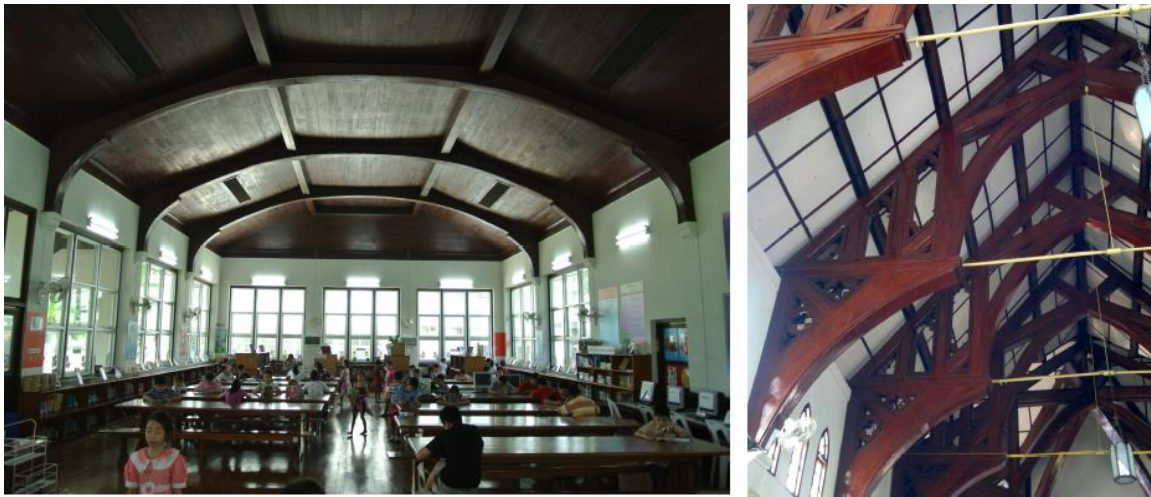
Figure 4: The inside of Power Hall (built in 1928), using the Wooden Rigid Frame Structure to maximize the width of the building. Today it functions as a library. [photos by Sant Suwatcharapinun]
