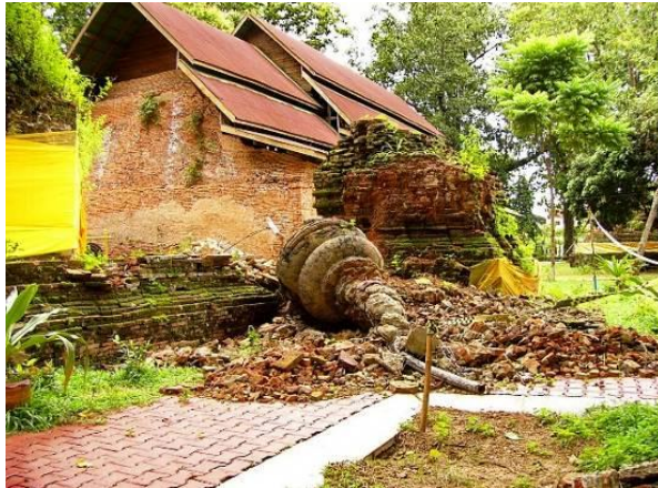
Figure 1: Wat Chediluang Temple in Chiang Saen, damaged by March 24, 2011 Earthquake.
