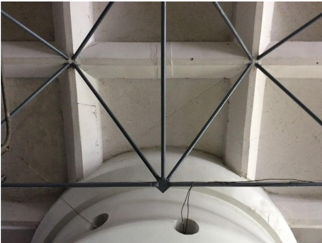
The underside surface of the concrete domes, while painted white, still allows the mark of bamboo-mattress to be partially visible
