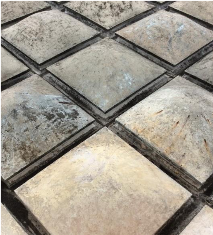
Roof concrete domes; each dome has a square base of 2.5 x 2.5 m. – the size that can readily be controlled by human hands.
